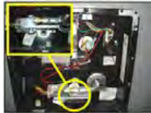
Water heater drain plug
