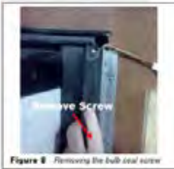
Figure 8 Removing the bulb seal screw
